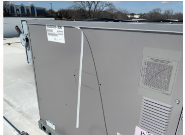
A few of the HVAC units may have some potential seal issues.
