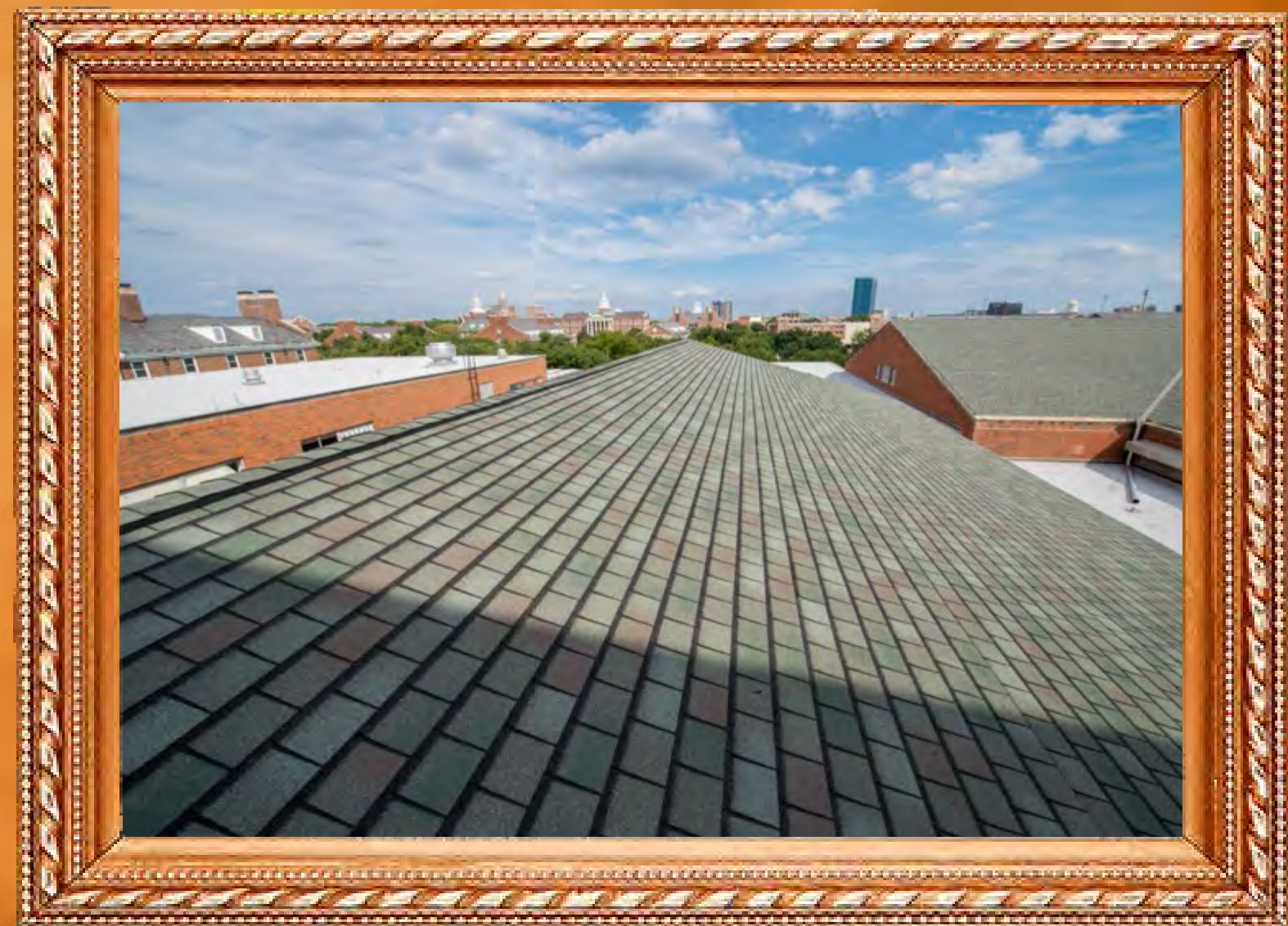
Remove & replace with GAF Slateline composition shingles
