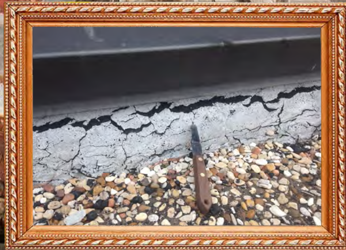
Existing coal tar pitch roof was improperly repaired causing pre-mature roof system failure
