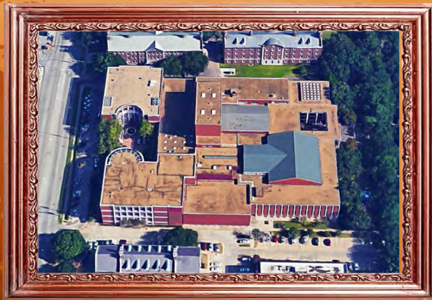
Before Re-roof Existing coal tar pitch
