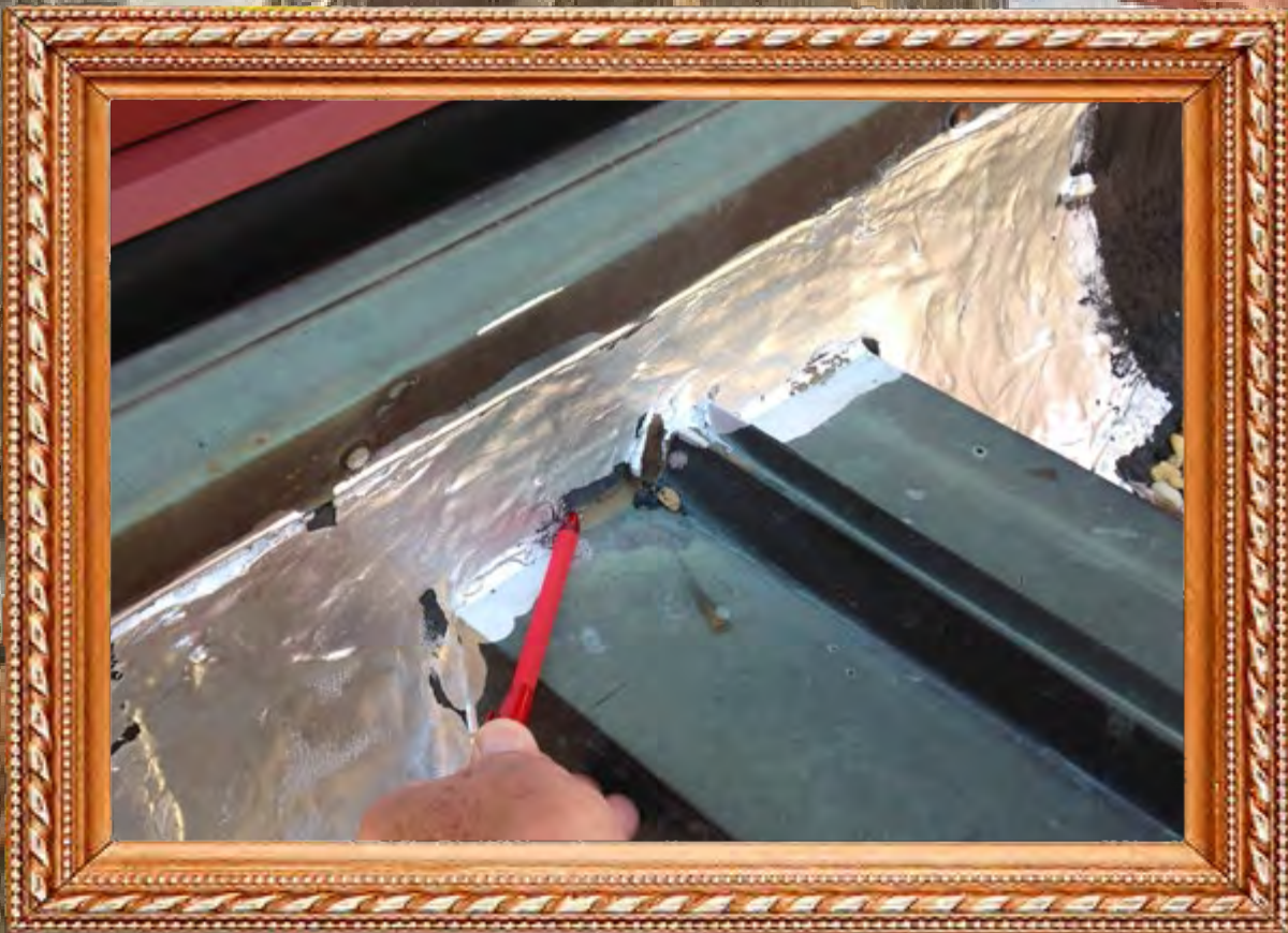
Existing coal tar pitch roof was improperly repaired causing pre-mature roof system failure
