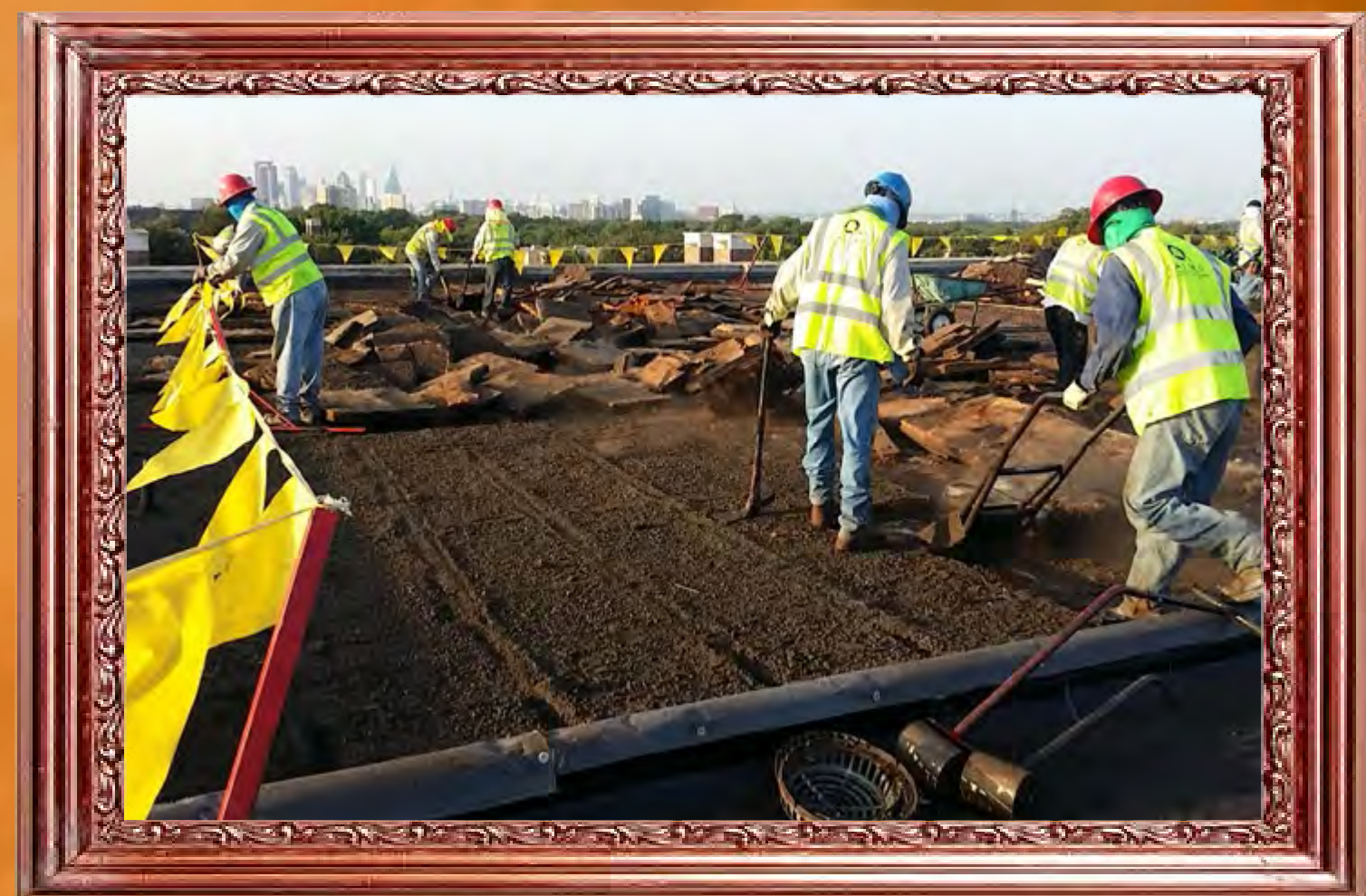
Removal of the phenolic insulation
