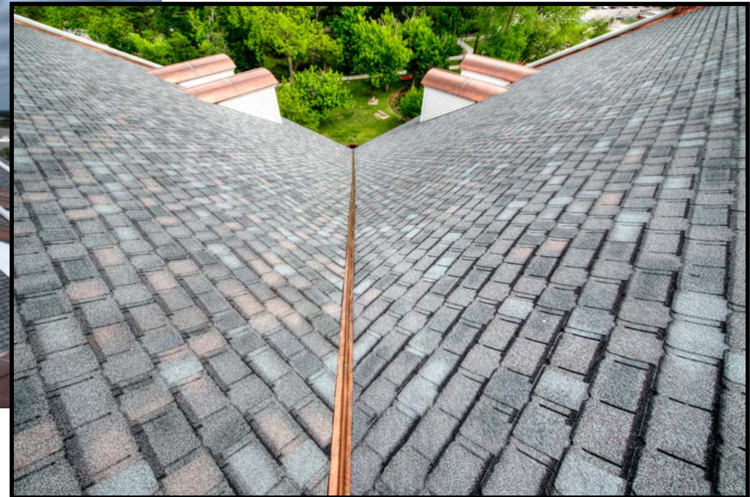
Composition Shingle Roof System — 44,735 SF on 9/12 roof pitch
