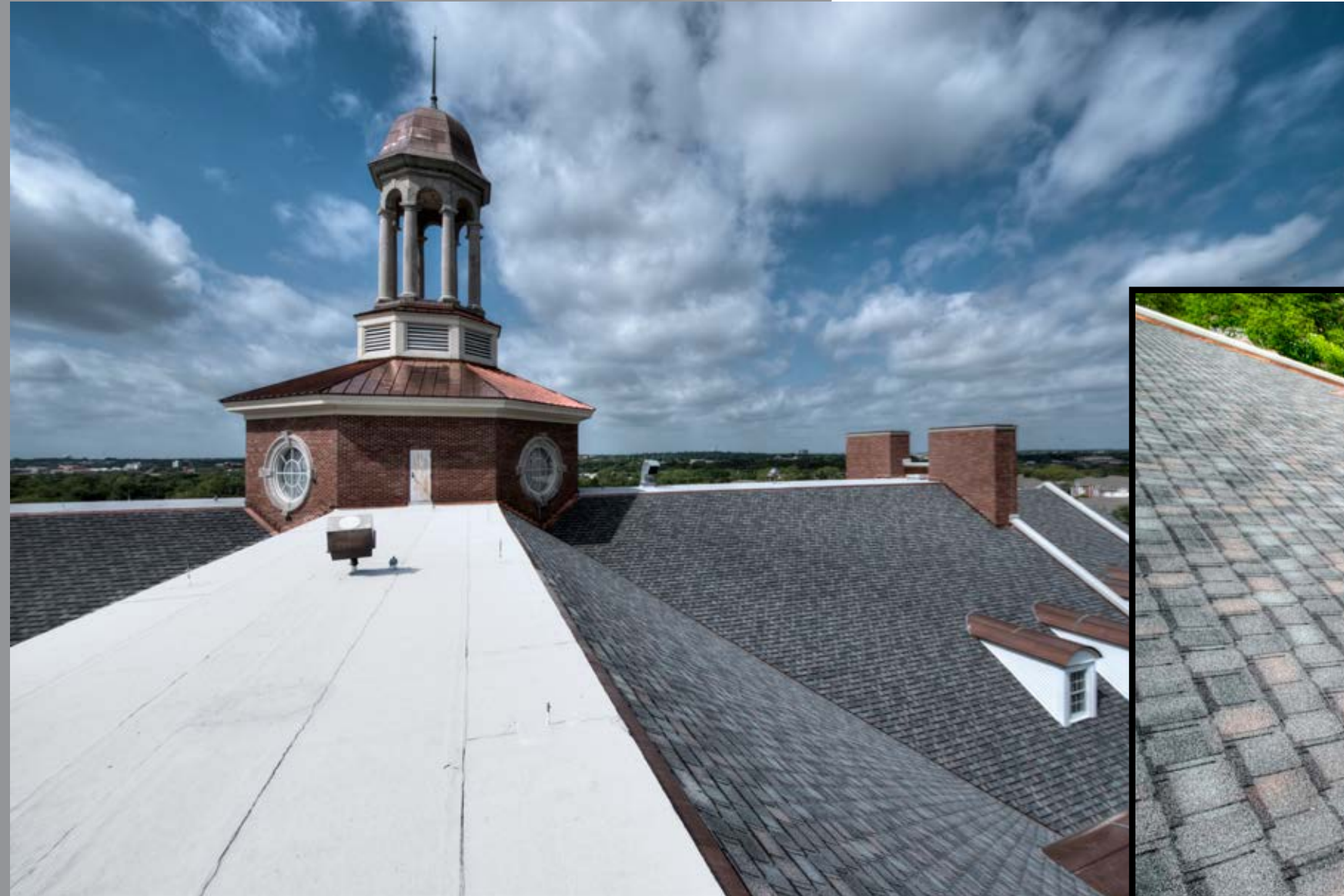
Modified Bitumen Roof System — 4,789 SF over four different wings
