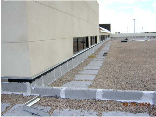
Progress: Walk pads at BUR.
