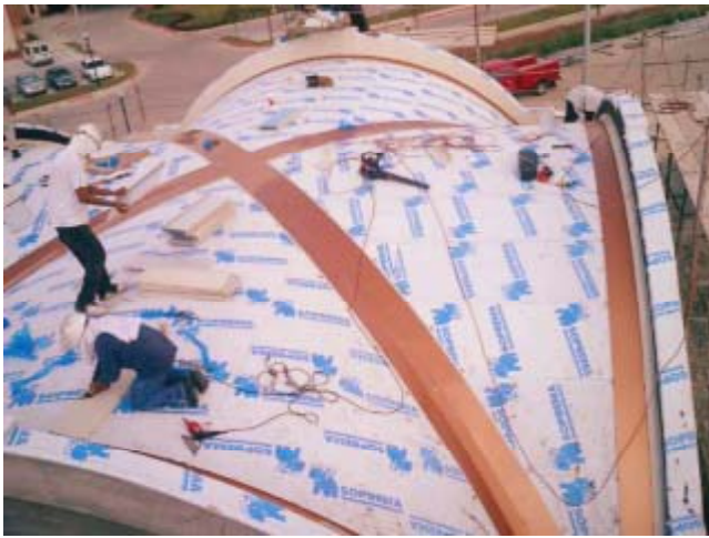
Progress: Layout of curbed metal valley with ice and watershield.
