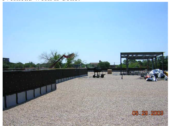
Progress: Overview of BUR system.
