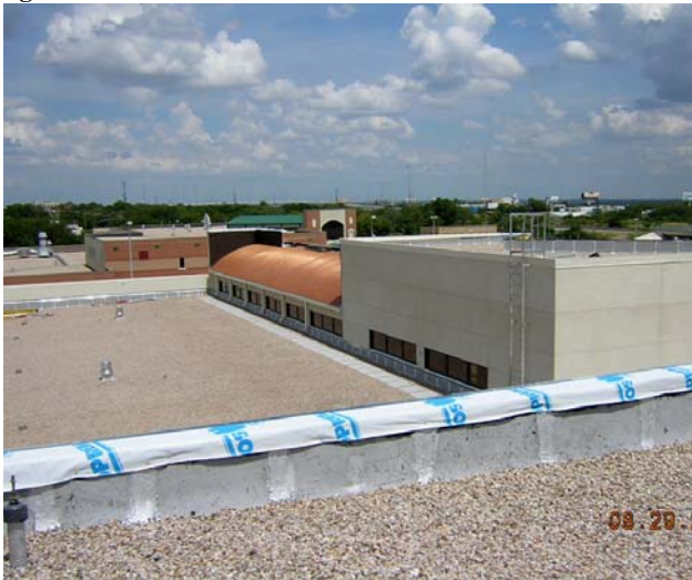
Progress: Multiple roof level and different roof systems.
