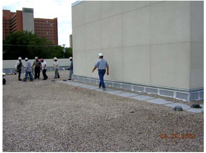
Progress: Walk pads at BUR
