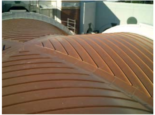
Installed System: Clay tile coping removed to permit ACM removal and new flashing membrane to over lap parapet wall..
