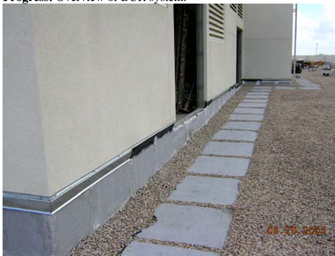
Progress: Walk pads at BUR.
