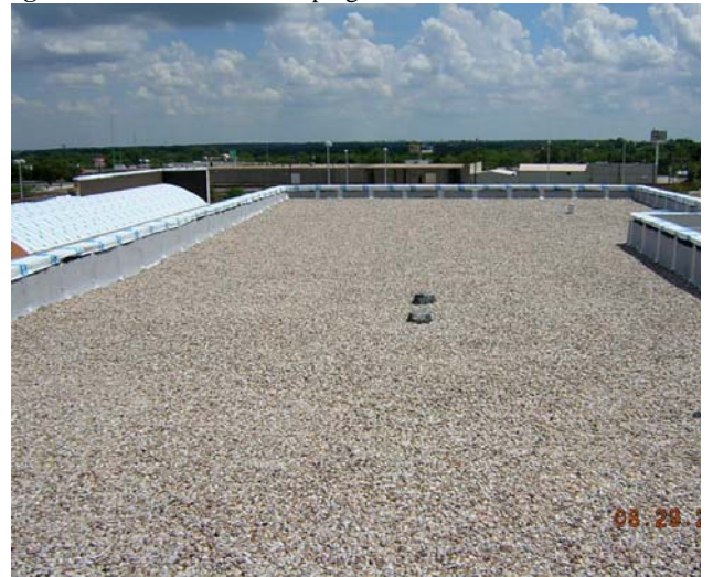
Progress: Overview of BUR system.
