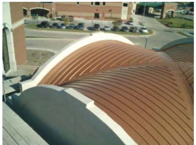
Progress: Safety lines and clay tile roof and modified membrane
