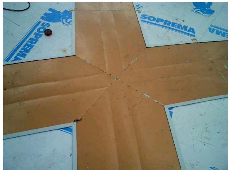
Metal Roof Valley Layout Pattern
