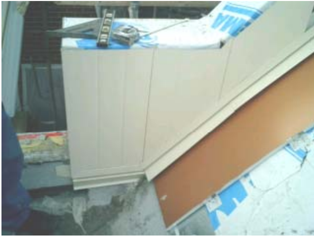
Progress: Curved metal roof termination against vertical wall surface.
