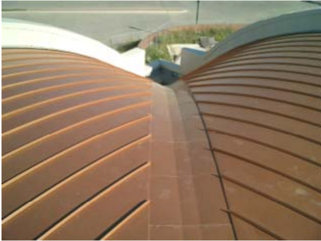
Progress: Curved metal roof termination against vertical wall surface.
