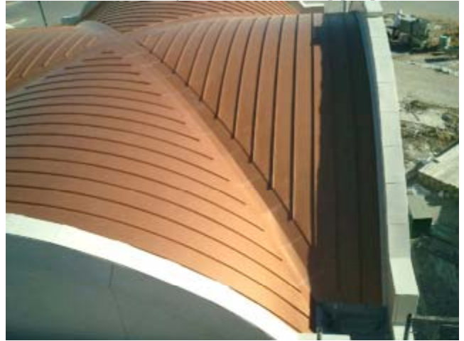
Installed System: Clay tile coping removed to permit ACM removal and new flashing membrane to over lap parapet wall..
