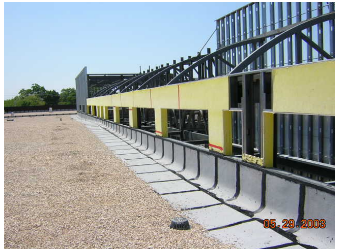
Progress: Gravel held back around walkpads until overhead work is done.
