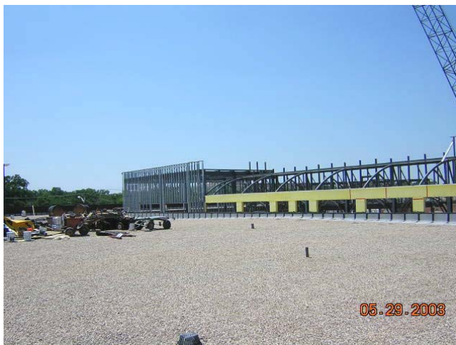
Progress: Overview of BUR system.
