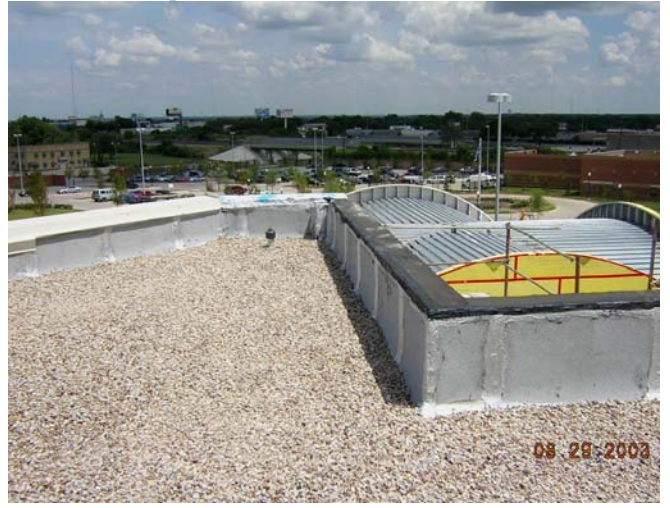
Progress: Unfinished metal coping.
