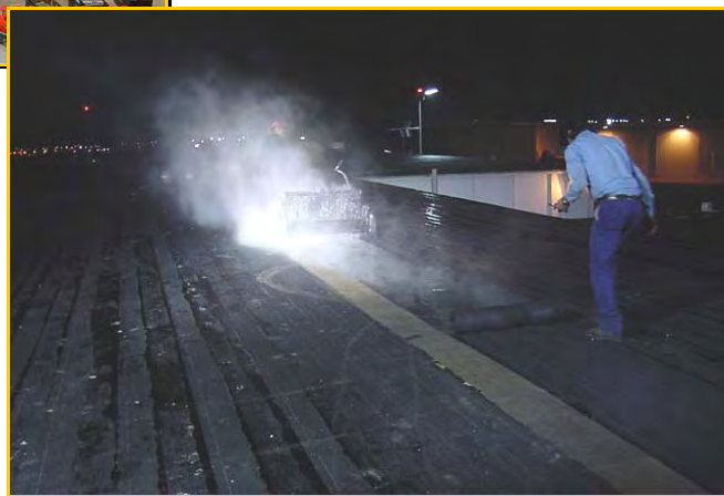
Work During The Night
