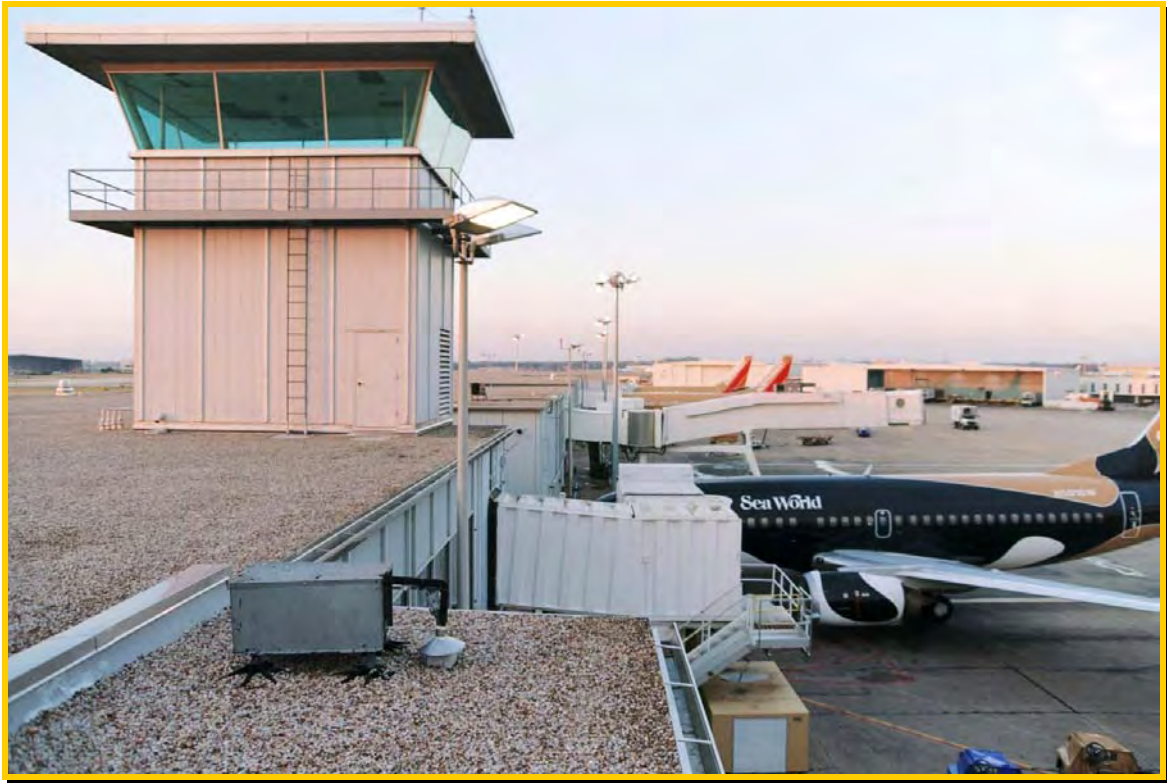
Planes Parked At The West Concourse Completed BUR
