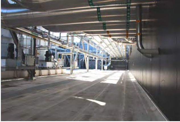
Energy Cap Modified Roof
