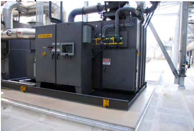
Energy Cap Modified Roof
