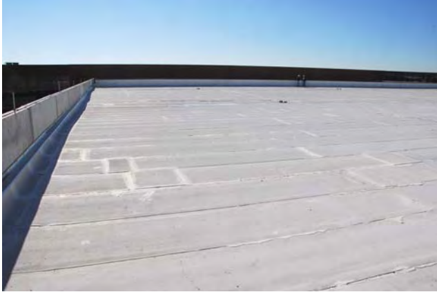
Energy Cap Modified Roof
