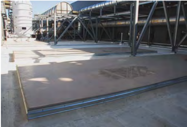
Energy Cap Modified Roof
