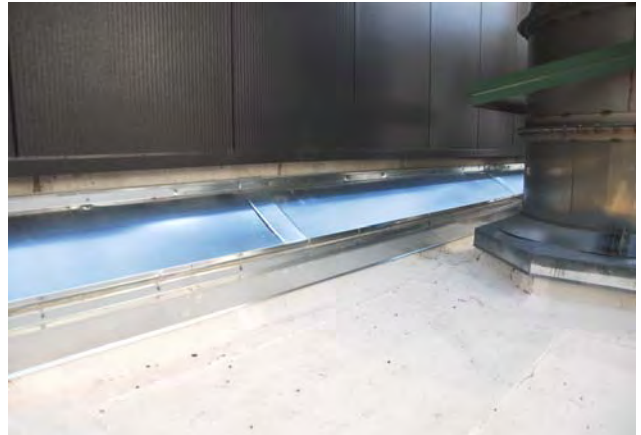
Energy Cap Modified Roof
