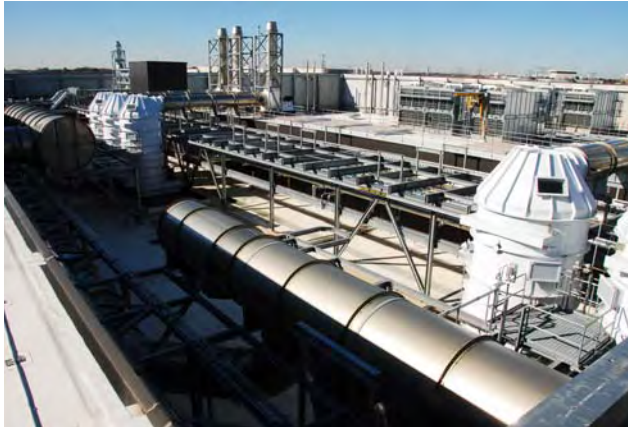
Energy Cap Modified Roof
