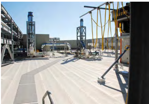
Energy Cap Modified Roof
