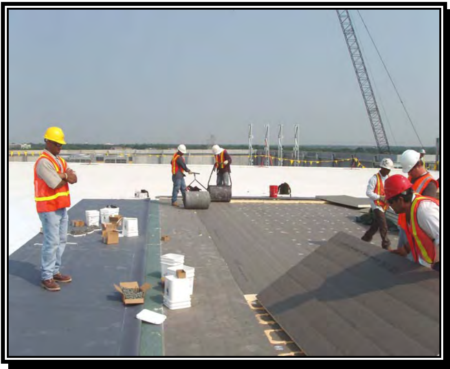
Installing the Multiple Layers of Insulation
