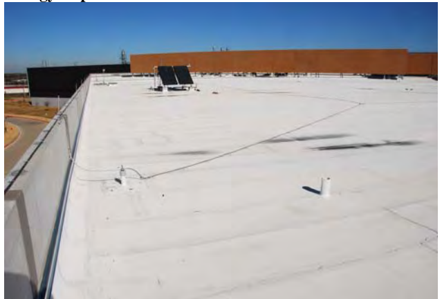
Energy Cap Modified Roof
