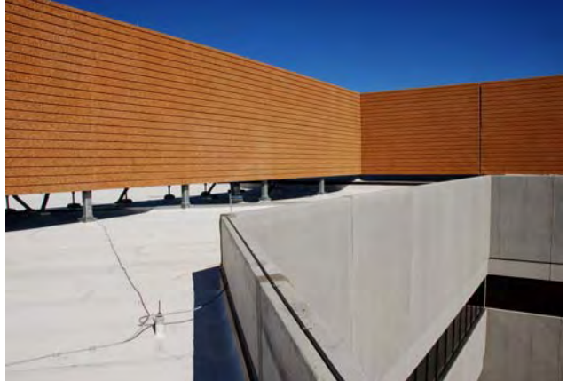
Energy Cap Modified Roof
