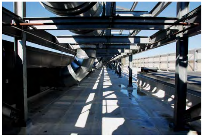
Energy Cap Modified Roof
