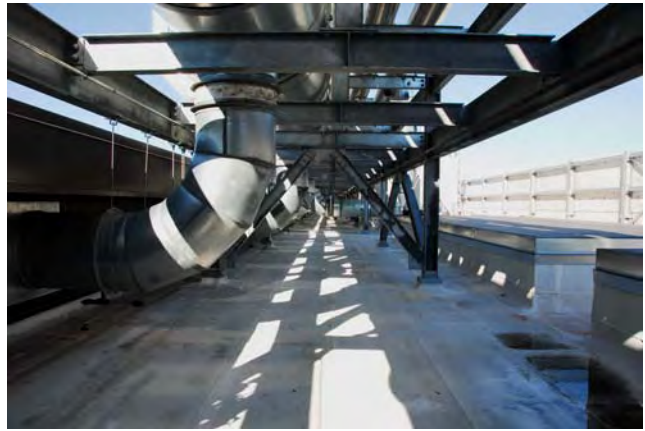
Energy Cap Modified Roof
