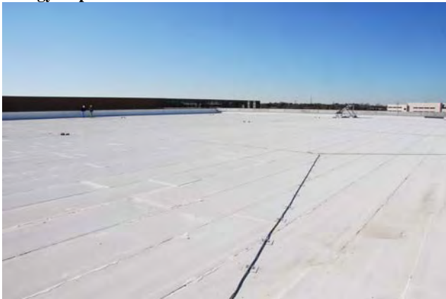
Energy Cap Modified Roof
