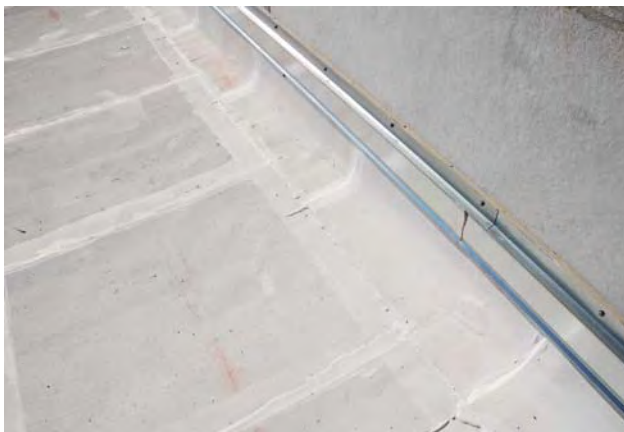
Energy Cap Modified Roof
