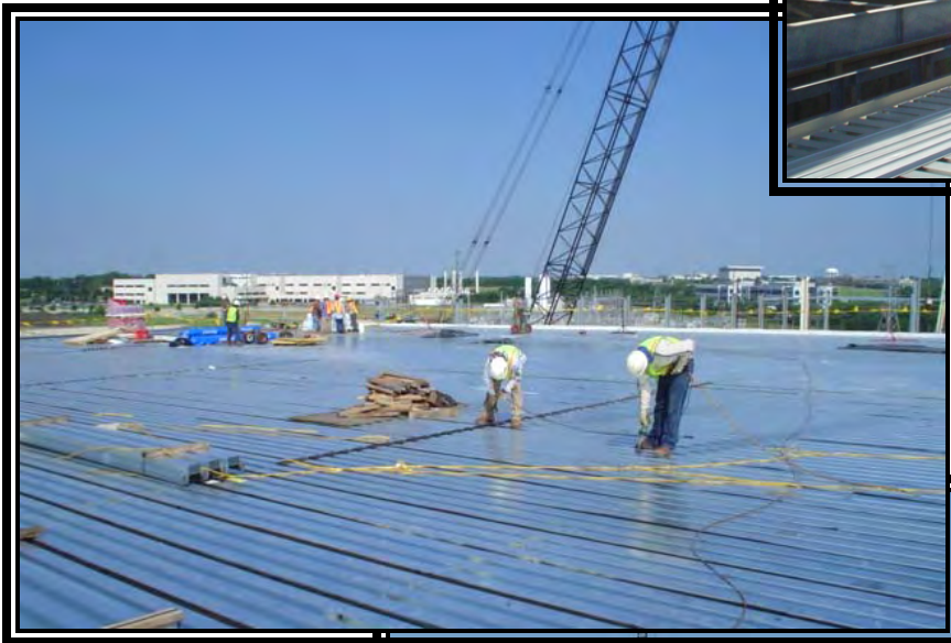
Installation of the Self-Adhering Membrane at Metal Deck End Laps, Side Laps and at Perimeter
