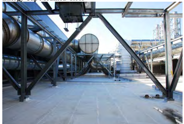
Energy Cap Modified Roof
