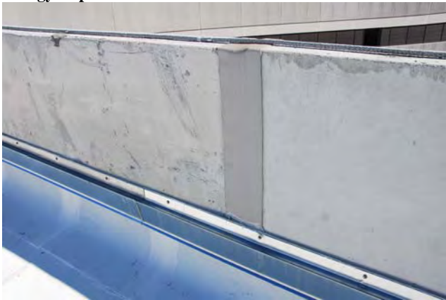
Parapet Joint Seal
