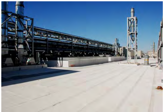
Energy Cap Modified Roof
