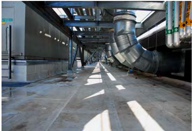
Energy Cap Modified Roof
