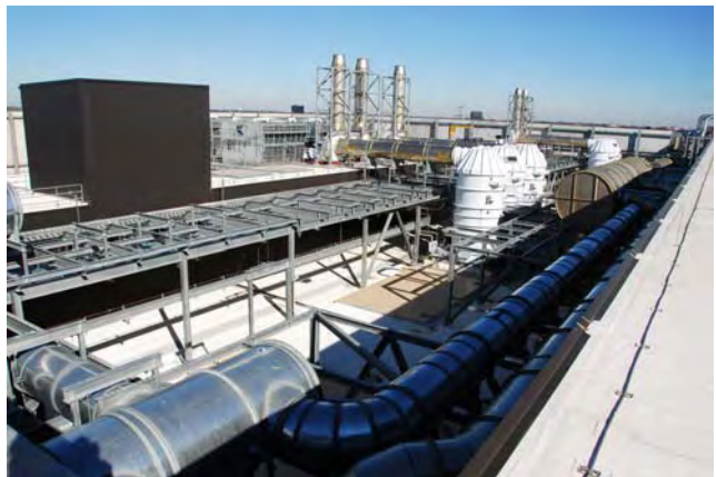
Energy Cap Modified Roof
