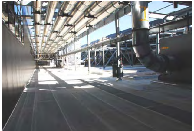
Energy Cap Modified Roof
