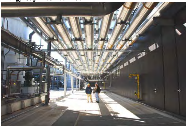
Energy Cap Modified Roof
