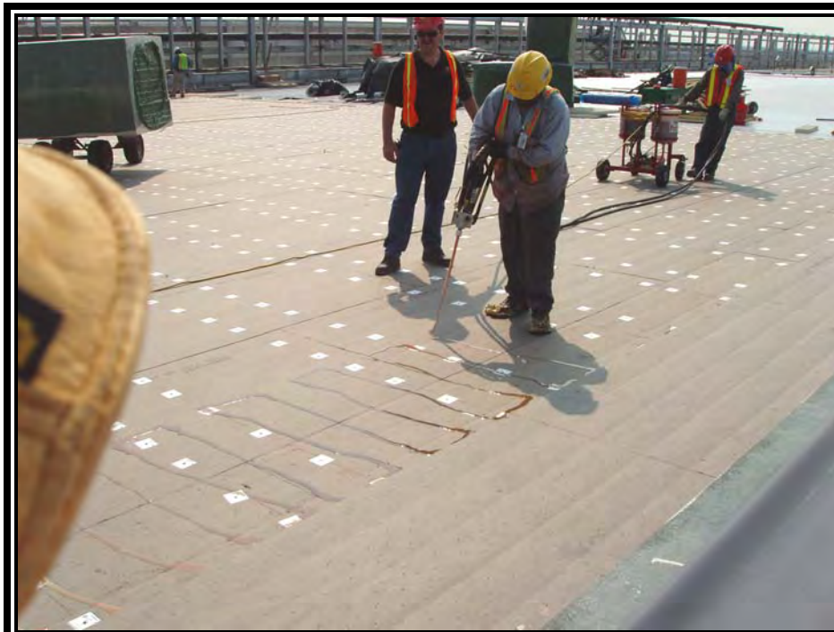
Crew Installing the Olybond Adhesive
