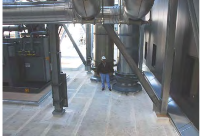
Energy Cap Modified Roof
