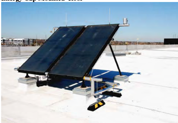
Energy Cap Modified Roof
