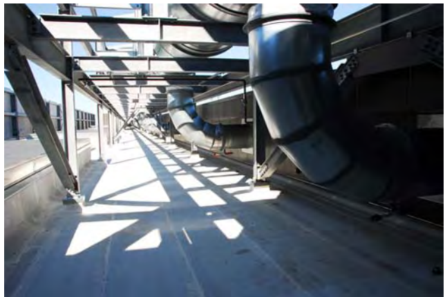
Energy Cap Modified Roof
