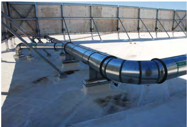
Energy Cap Modified Roof
