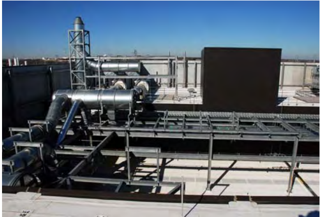
Energy Cap Modified Roof
