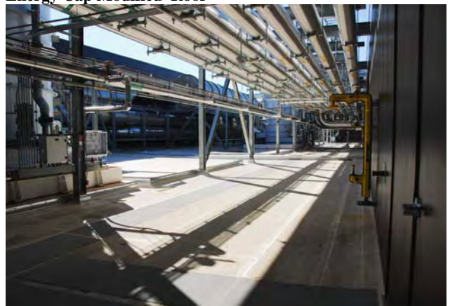
Energy Cap Modified Roof
