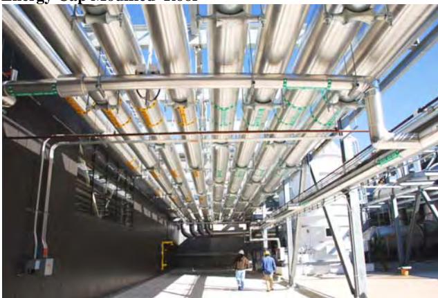
Energy Cap Modified Roof
