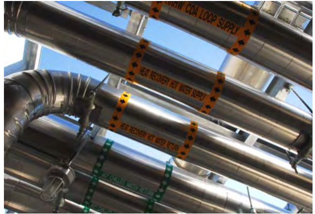
Energy Cap Modified Roof
