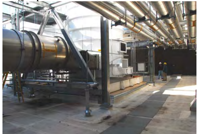
Energy Cap Modified Roof
