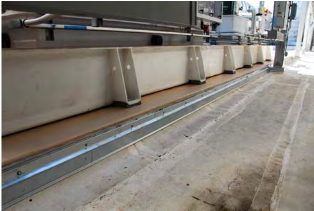
Energy Cap Modified Roof
