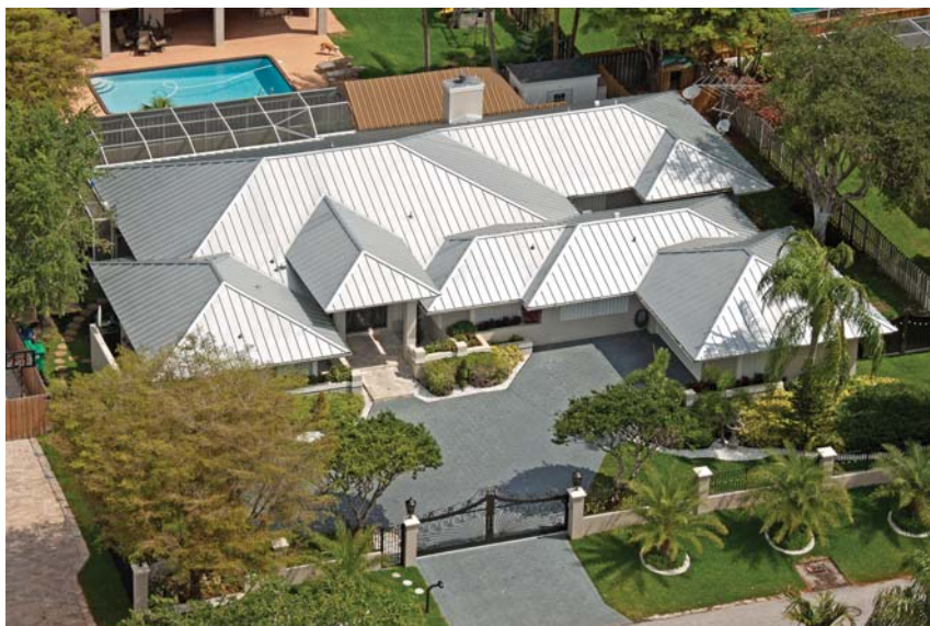
Istuea Roofing photo
