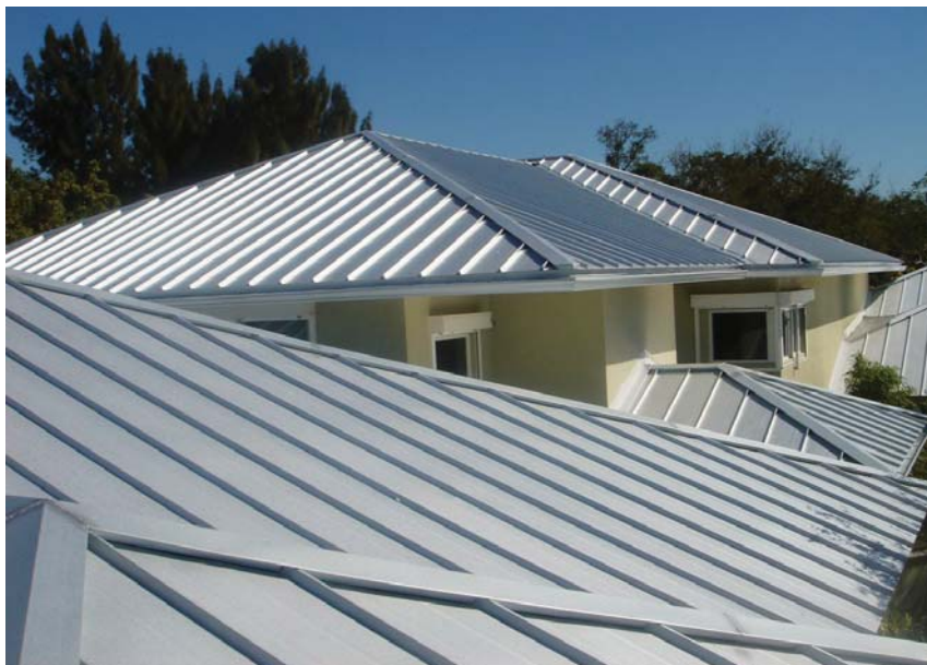
Istuea Roofing photo
