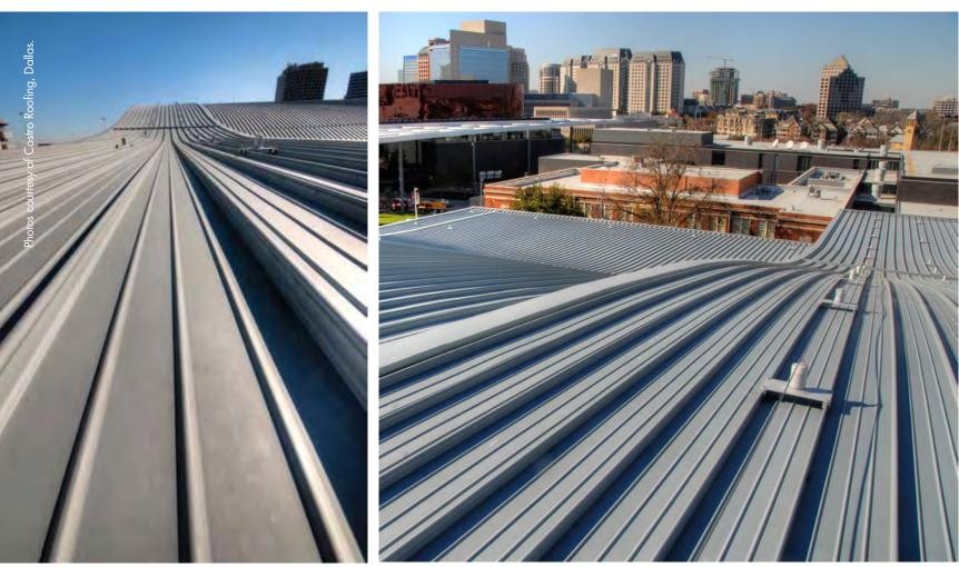
The Dallas City Performance Hall's roof system incorporated the longest Kalzip® single-length, roll-formed mechanically seamed AluPlusZinc panels in North America.
