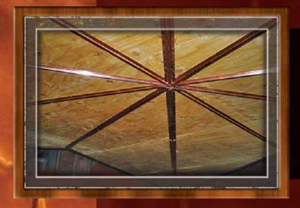
The star's frame is held together by a strong brace system that protrudes through the exterior of the ceiling and through the outside deck.
