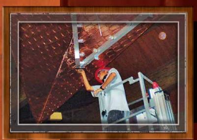
The star's exterior frame was wired and bulbs were installed before the secondary lit star was put in place.
