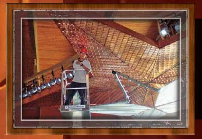
The outside of the wooden and metal frame was covered with stamped copper shingles that were meticulously placed at a 45 degree angle.
